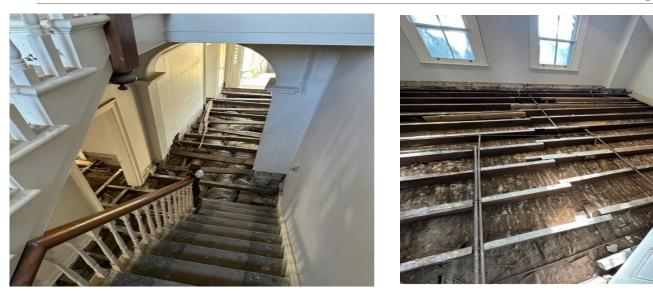
Whilst the floors were up, Tony had plumbers removing old redundant gas heating and making the under floors safe. Electricians also ran cables extending GPO (power point) cables as new skirting boards will be installed.
